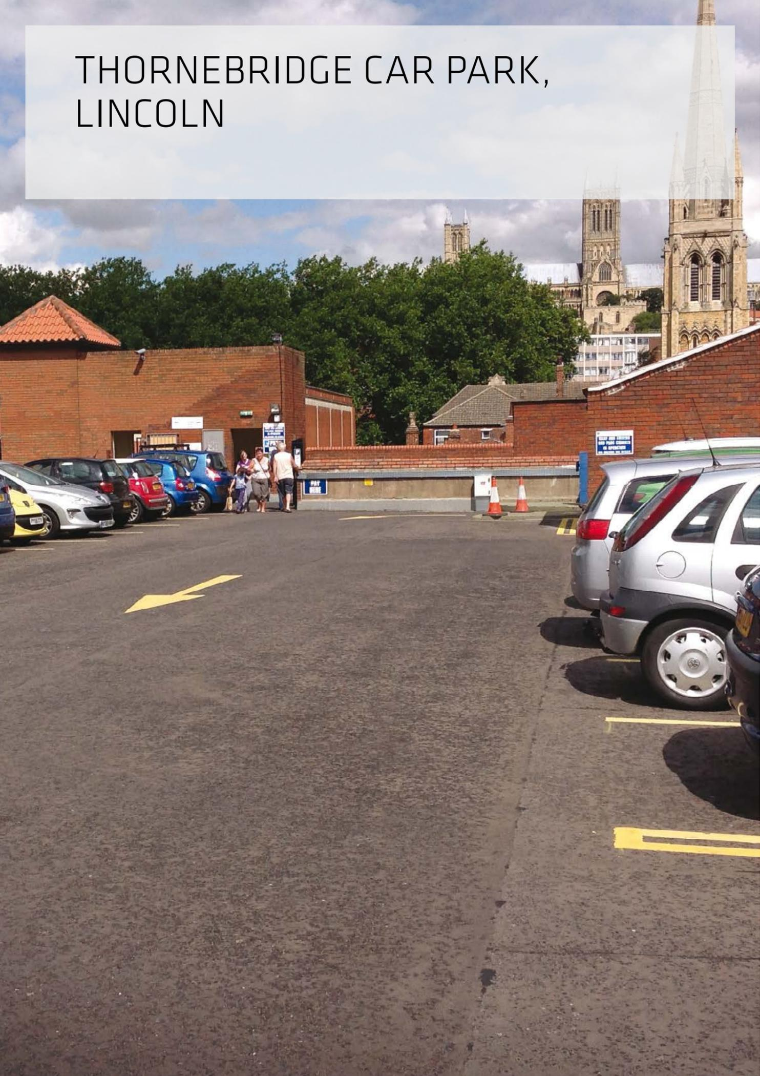
**SIKA'S BRIDGE DECK WATERPROOFING SYSTEMS** were used on Thornebridge car park in Lincoln, as it was in desperate need of renovation with a failing asphalt decking system and no waterproofing membrane.
