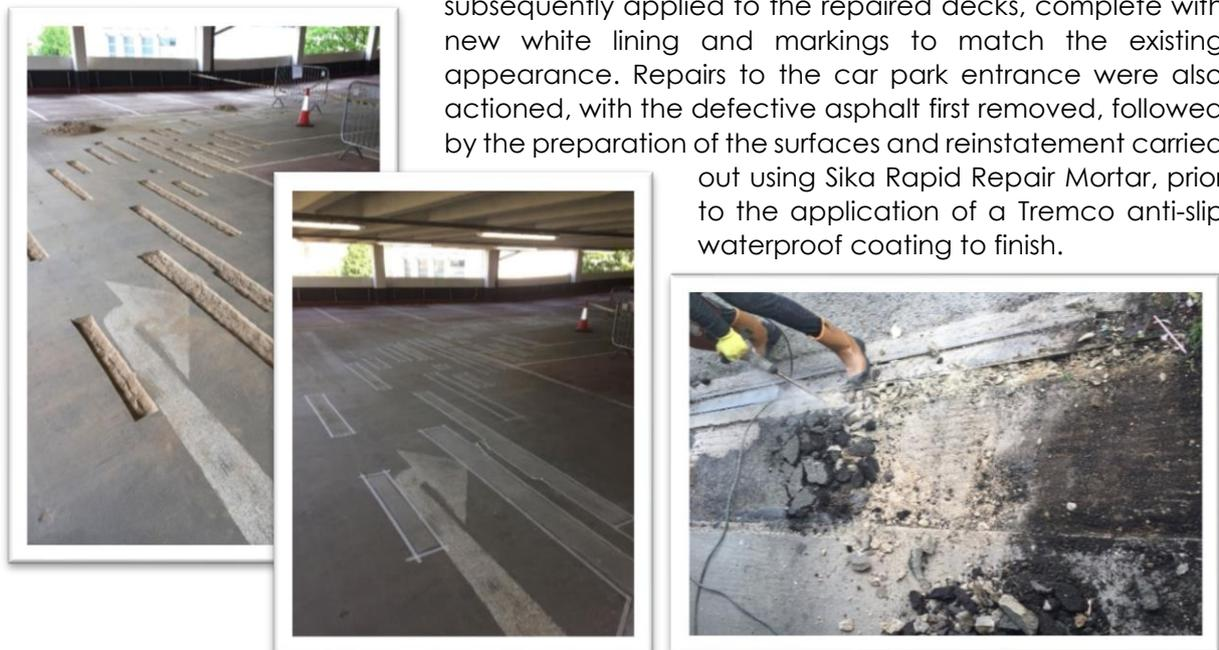
**The outcome:** With all concrete defects to the car park decks and entrance slabs repaired, the defunct cathodic protection system removed and with the addition of the new anti-slip deck waterproof system, the car park structure was protected from further degradation for the foreseeable future. The works completed by **APA** ensured the Mayorhold Multi-Storey Car Park was successfully refurbished and was promptly returned to its full capacity.
