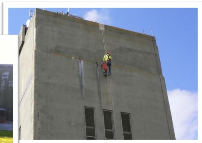
**The outcome:** Both structures within the RAF Leeming station were remediated against all areas of cracked and spalling concrete, with any leaking cracks chased out and filled, before completing the roof repairs. The application of a guaranteed reinforced waterproof membrane to both rooves ensured further protection against future leaking, damage and corrosion, providing a long-term solution for the MoD.
