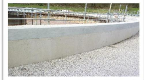
**The outcome:** The concrete walls to the two PSTs were successfully re-profiled, with the tops of the walls provided with a level running surface with an anti-slip finish as had been desired by the Client (YW). The protective coating system added increased durability to the repaired wall tops and increased the service life of the tanks thereby reducing future 'life cycle' maintenance costs.
