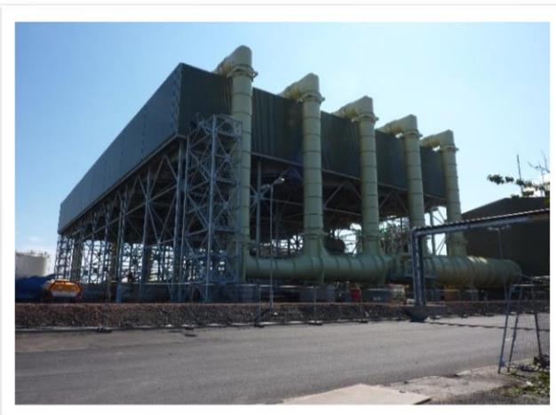
**The solution:** **APA** provided a survey & investigation proposal including testing for the presence of HAC and chlorides, as well as testing for carbonation and surveying for defects. The site team completed the works safely and within a strict time frame to suit an already congested programme of works during a planned outage. Access was achieved using Mobile Elevated Platforms (MEWP) under the strict control of trained banksmen.
