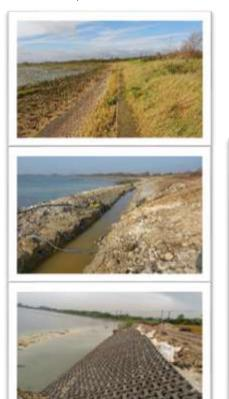
against future coastal erosion. Where possible, previously removed and preserved materials, including the Armorloc blocks, were re-used in order to reduce wastage and maintain the client's budget. The refurbishment works resulted in a significantly improved appearance to the embankment, as well as a durable coastal defence structure.
