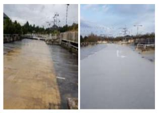
drainage pipes/gullies were installed to the base of the ramps. The entire top deck coating of each carpark was removed, hybrid galvanic anodes were installed to each area where high chlorides had been identified, and the deck surfaces were coated with a Tremco MMA Flexible Waterproof System. The perimeter gutter system of the office buildings were re-lined with a liquid applied waterproof system and expansion joints and plasterboard ceilings were replaced.
