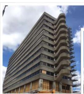
external concrete repairs and apply protective coatings to the surrounding elevations of this 13-storey building over the Summer of 2018, prior to the increased student demand for housing accommodation.
