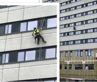
**The outcome:** The refurbishment was completed in September 2018, just in time for the start of the new academic term. All external defects were closely identified and addressed, allowing for the effective application of protective coatings, which will guarantee prolonged prevention from future deterioration. The use of the specialist roped access technique also allowed for the
