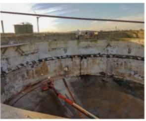
**The solution:** Initial works consisted of various surveys and tests to determine the scope of remedial works required, including structural surveys, carbonation tests and chloride profiling. Upon completion of testing, internal concrete defects located on both tanks were identified, broken out and repaired using a high strength, polymer modified SikaMonotop 612 repair mortar, complete with the provision of protective coatings. External concrete surfaces were
