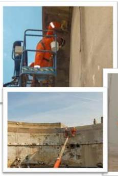
then thoroughly prepared prior to the application of a SikaMonotop 620 to infill any honeycombing and blow holes. A fairing coat and Sikagard anti-carbonation coatings were then applied as protective finish coats. Additional works included the coating of the internal top bands of both tanks with a hot sprayed polyurea lining, to provide further long-term protection.
