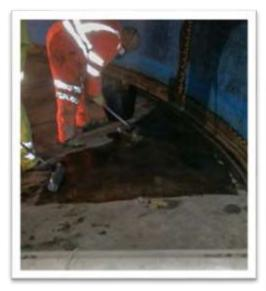
application of a Sikalastic 841 Hot Sprayed Polyurea Waterproofing System, complete with a tack coat primer.
