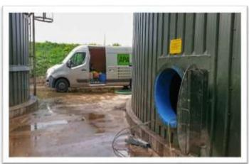
**The outcome:** The works within the primary digester tank were completed within a one-week period, ensuring minimal disruption to the plant's daily activity. The choice of iron silicate propelled abrasive blasting allowed for surface cleaning without excessive particle breakdown, minimising the quantity of dust generated during the works, and the provision of
