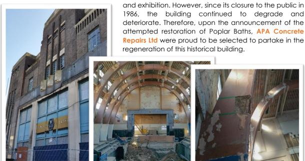
**The solution:** APA were contracted to design and install an impressed current cathodic protection system (ICCP) to masonry clad structural steel framed elements at Poplar Baths. Brick masonry was sympathetically removed to allow for the installation of the ICCP system
