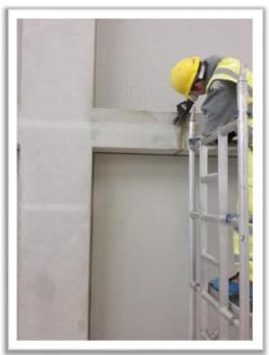
struck" finish. The targeted areas primarily encompassed repairs to internal concrete surfaces, including surrounding walls as well as the walls of the lifts and stairs.
