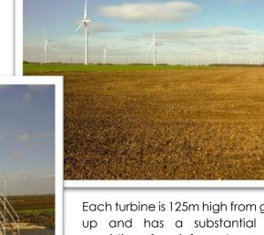
Each turbine is 125m high from ground level up and has a substantial foundation consisting of a reinforced concrete ground base cast on top of a series of piles driven deep into the ground. The foundations are subjected to considerable force over their lifecycle from wind loadings, therefore it's crucial that each base remains in serviceable condition.
