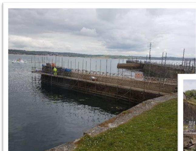
overlay of the full areas of the wall using a spray applied concrete at a thickness of 50mm, finished with a steel float to provide a smooth finish.
