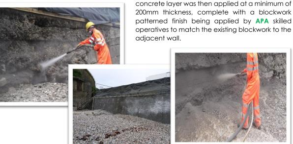
**The outcome:** Being the most efficient method of concrete application, the process of spray concreting the Southern face sea wall was completed in August 2016, ensuring this everpopular destination could be promptly re opened to the public. The materials used for the
