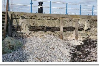
**The solution:** The surface of this Southern faced seawall was first prepared by the removal of the timber fenders along with any redundant metal fixings, followed by the removal of any loose fill material using mechanical breakers and a process of high-pressured water jetting. Once a suitable key for repair was created, deep pockets within the wall were reinstated back to the original profiles prior to fixing two layers of steel wrapping mesh to the wall. A sprayed
