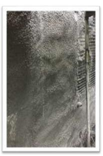
The outcome: The concrete repairs to the retaining wall on Clints Road were completed by September 2017. The 'weep pipes' installed had the resulting effect of the alleviating potential water build-up, arresting its deterioration and providing a stable foundation for the walling
