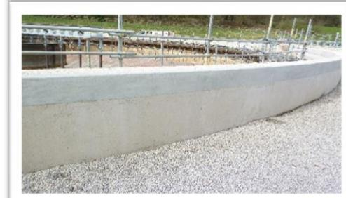
**The outcome:** The concrete walls to the two PSTs were successfully re-profiled, with the tops of the walls provided with a level running surface with an anti-slip finish as had been desired by the Client (YW). The protective coating system added increased durability to the repaired wall tops thereby increasing the service life of the tanks thereby reducing future 'life cycle' maintenance costs.
