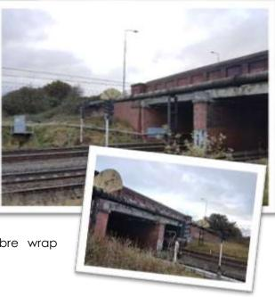
to undertake concrete repairs and a carbon fibre wrap containment to the bridge soffits.
