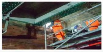
**The outcome:** The repair and strengthening works to the soffits of Golborne Railway Bridge were completed despite repeat interruptions from train movements as well as numerous possession cancellations, and the risk of sections of concrete falling onto passing trains was mitigated throughout.
