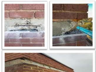
**The solution:** Specified areas of defective concrete were first marked out and subject to saw cutting and breakout, before exposed steel reinforcing was cleaned and protected using Fosroc Nitoprime Zincrich. Fosroc Nitobond HAR was then applied to the prepared concrete substrate, prior to applying Fosroc Renderoc HB to reform the defective concrete, with the finish ensured to
