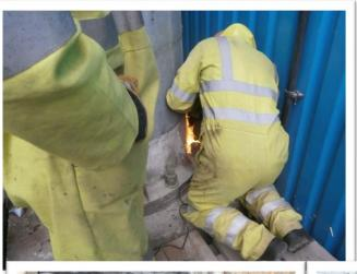
form the original concrete profile, before a new stiffener plate was welded to the existing corroded stiffener. completion, the exposed steel was coated to provide additional weather protection.
