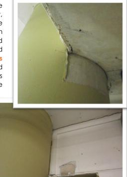
**The solution:** The surfaces of eight of the concrete columns which supported levels 10 and 20 of the car park were first prepared through a process of grit blasting. Once the resulting dust
