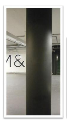
thereby creating minimal disruption to the centre's everyday activity. Due to the carbon fibre composite strengthening completed by APA, the reinforced columns, complete with the added assurance of two hours fire resistance, provided the increased load carrying capacity to enable the additional floor level to be constructed.
