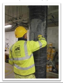
gn a process of grit blasting. Once the resulting dust and debris had been removed, any identified defects in the columns were repaired and cured. A Sikadur resin was then applied to the substrate before a Sikawrap stressed carbon fibre fabric wrapping was cut and applied to each of the eight columns, with this process being repeated until each column was encased with the desired number of protective layers.
