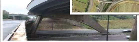
**The solution:** APA Concrete Repairs Ltd were involved in refurbishing the supporting structures as part of a central barrier replacement scheme on the M1 section. An extensive programme of concrete repairs was completed during limited night and weekend lane closures. These works included breakout by hydro-demolition, rebar replacement, installation of galvanic sacrificial anodes, waterproof coatings and included the provision and maintenance of our own scaffolding access.
