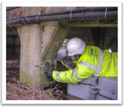
**The outcome:** The various surveys and testing carried out resulted in the generation of a report, detailing the findings of the defects survey, laboratory analysis and results, as well as recommendations for concrete repair and remedial works. Following completion of these surveying and testing works, Timsbury Bridge underwent a concrete repair and refurbishment programme.
