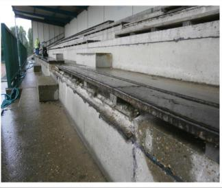
**The outcome:** The repair works undertaken to Wimbledon athletic stand were completed in August 2015 and resulted in the structural reinforcement and integrity of the four staircases which run through it. The galvanic anodes installed additionally provided the guarantee of prolonged protection against future corrosion, further increasing the life cycle of the repairs.
