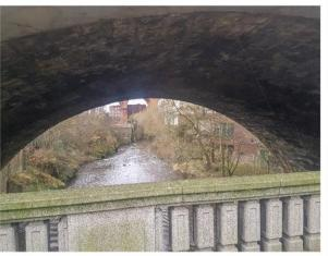
**The solution:** Prior to the concrete repair programme, existing coatings were first removed via scraping and washing, in order to provide a sufficient key for repairs. A hammer test was undertaken to the shotcrete render covering the arch intrados before a cementitious repair material was applied to failed areas of exposed brickwork.
